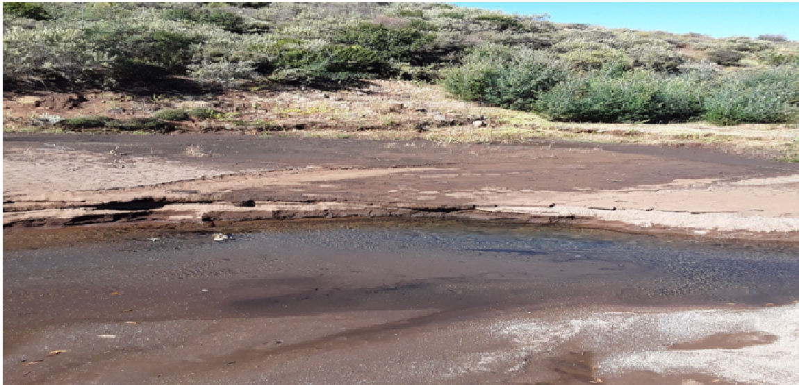
Fig. 4. Sedimentation in a community reservoir at Ha Mahloane, Bolahla
